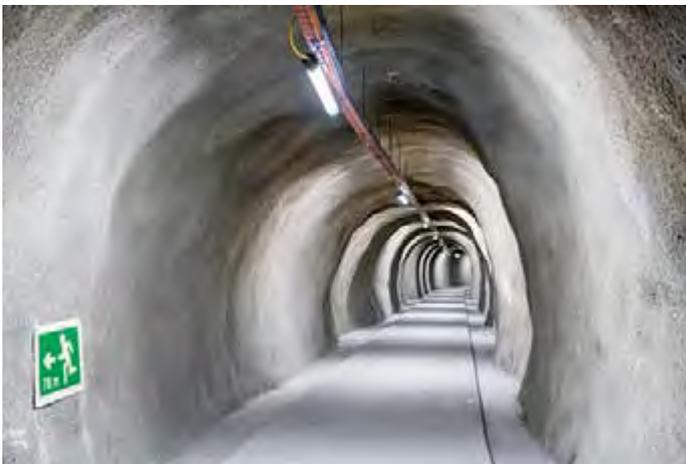
Following its general renovation, the 500 m long Schallberg tunnel can be seen in a new light. The luminaires were developed by the Swiss tunnel lighting specialists Rigamonti and equipped with LED components from Tridonic. The result is high-performance lighting system that offers an unprecedented of visual comfort and has a positive effect on overall feeling of safety among vehicle drivers.
